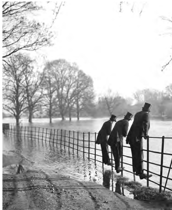
WATER WORLD Eton College, flooded here in the 1930s, has Old English roots meaning “river settlement.”
